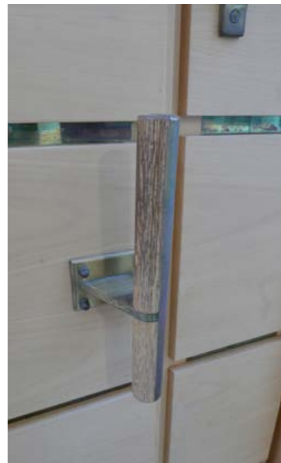
Istuntosalin oven puumessinkivedin.
