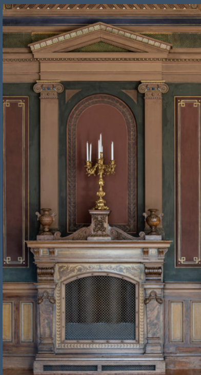
The wooden cabinet structure in the Bourgeois Hall conceals ventilation and heating equipment. Photos by Arno de la Chapelle.
