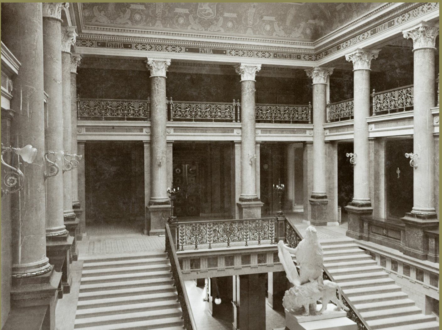
An early picture of the original colours and ornaments around the main staircase landing. The high-gloss lacquered faux marble columns are made of bricks while the landing floor structures are brick vaults supported by steel bars. The material initially intended for the flooring was limestone, but this was replaced by a novel, locally produced material: terrazzo. The decorative railings and handrails were cast at Högfors ironworks in accordance with Nyström's design. The first plaster model of Walter Runeberg's statue 'LEX' stands at the centre of the staircase. 1890s, Helsinki City Museum.
