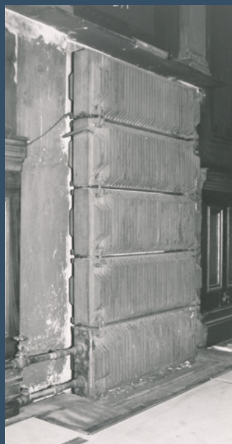
The steam radiators in the big assembly halls were hidden inside ornate wooden cabinets that resemble a mantelpiece. In the picture on the left, taken during the 1988 renovation, the cabinet has been removed revealing the original radiator. The picture on the right is from 2017. Pictures by Helander-Leiviskä Architects and architecture firm Okulus.
