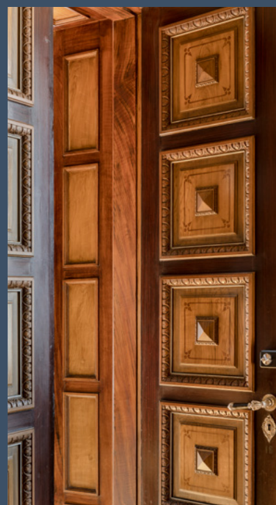
The doors of the assembly halls are the most magnificent and hierarchically significant in the building. The ensemble, which appears to be made of noble wood, consists partly of stained and lacquered oak and partly of painted and wood-grained pine, plaster, or stucco.
