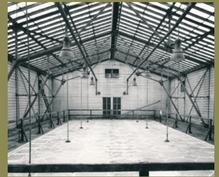
The iron frame of the glass ceiling above the main staircase is remarkably slim and delicate. This structure has remained mostly untouched throughout the decades and is a cherished feature of the building. Picture from 1979 by Veikko Laine, Finnish National Board of Antiquities.
