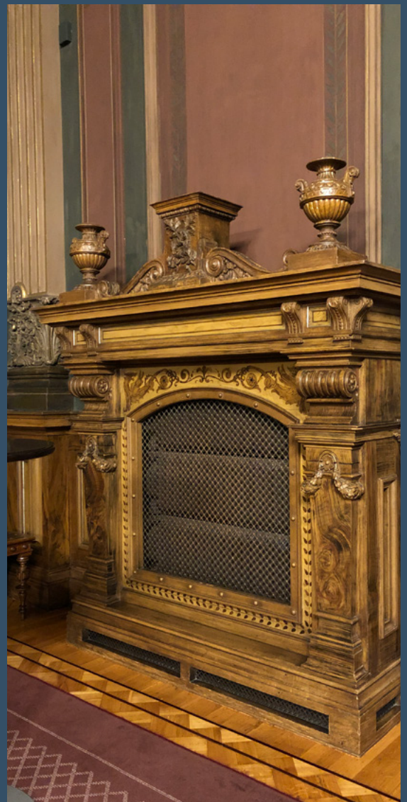
The steam radiators in the big assembly halls were hidden inside ornate wooden cabinets that resemble a mantelpiece. In the picture on the left, taken during the 1988 renovation, the cabinet has been removed revealing the original radiator. The picture on the right is from 2017. Pictures by Helander-Leiviskä Architects and architecture firm Okulus.
