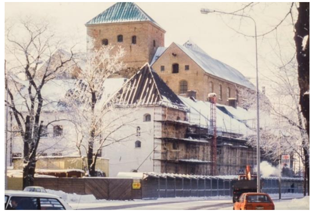
Picture 2: The bailey gets a new plastering (Kotkas 1985).
