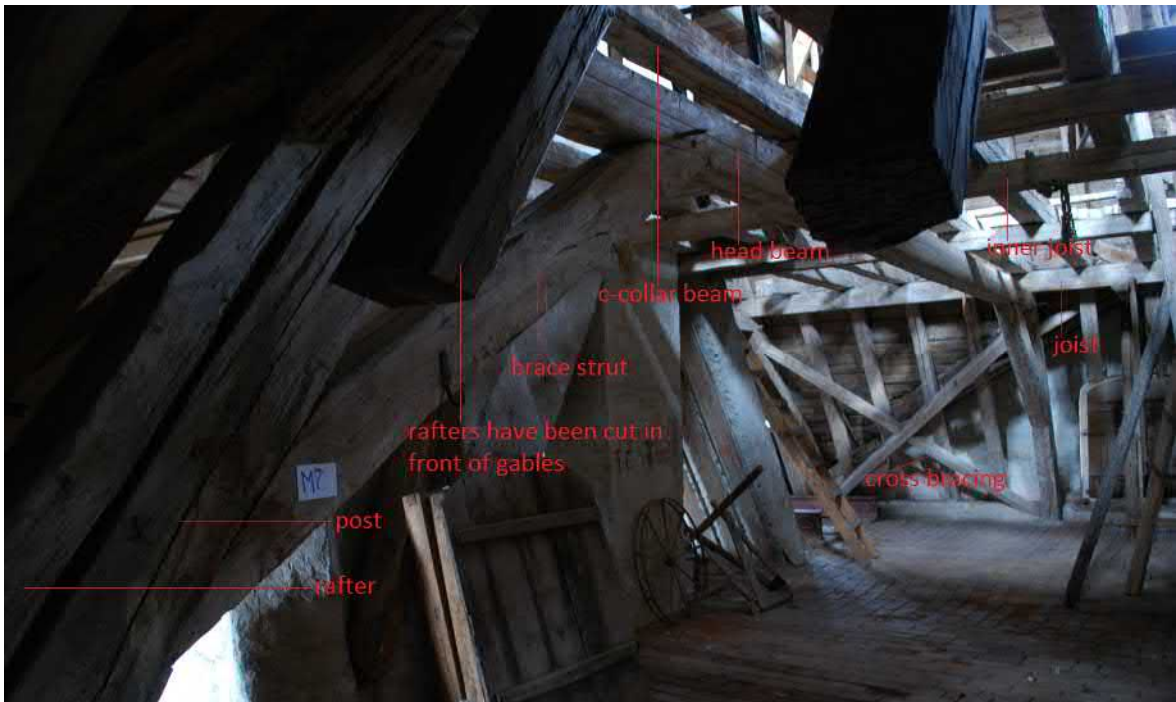
Figure 20. Leaning trestle spanning across between the long external walls.
