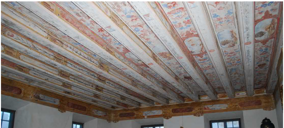
Figure 25. The ceiling of banqueting hall with original decorative paintings painted on the tie beams and bulkhead boards.
